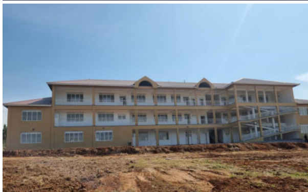
Complete building for the Faculty of Nursing and Health Sciences in Ruharo
