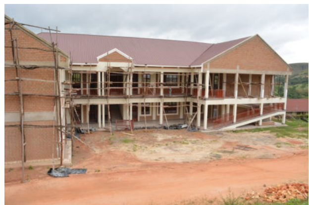
Interlocking Stabilized Soil Blocks (ISSB) building under construction
