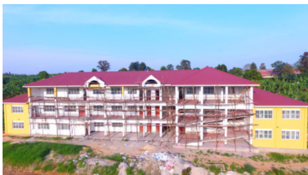
Ruharo School of Nursing under construction
