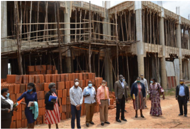
Science Laboratory Block underconstruction
