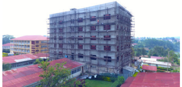
University Library expansion underconstruction
