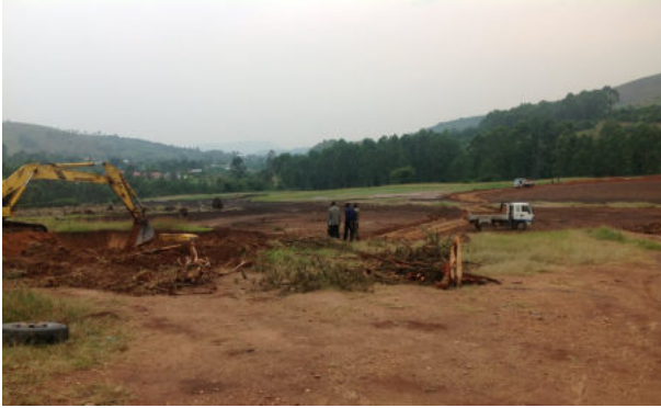
Leveling ground for Riverside sports complex
