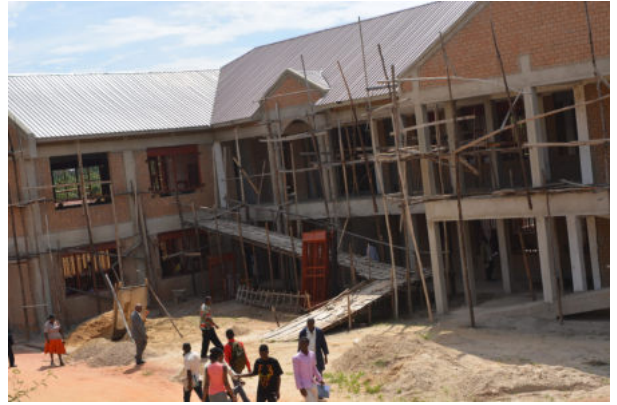
ISSB Building for the Faculty of Education underconstruction
