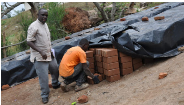
Estates staff operating an interlocking bricks making machine
