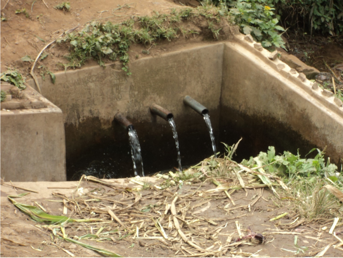
Plate 5. A protected water spring with three barrels. Note the clear water and the varying flow volumes in the different pipes
